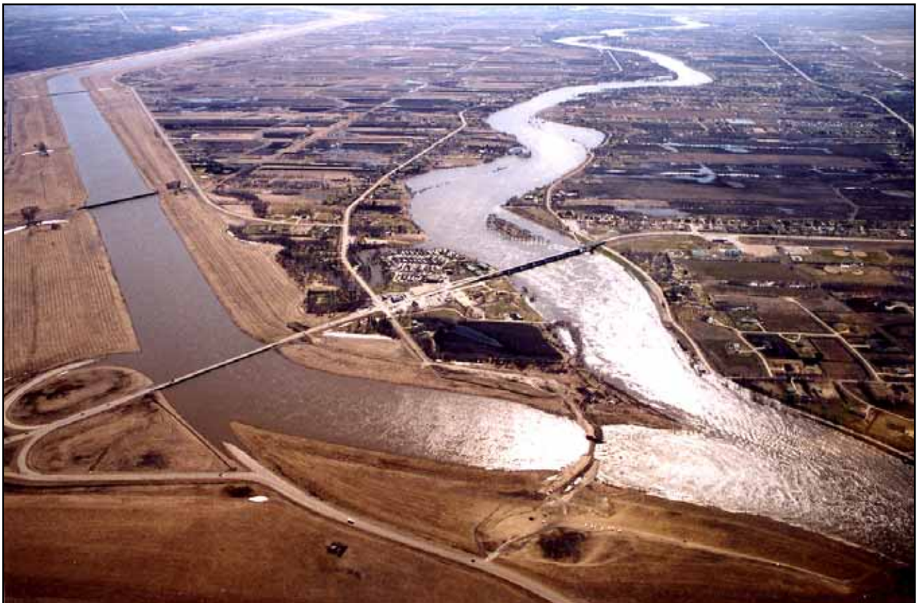
Floodway Exit at Lockport, 1997
