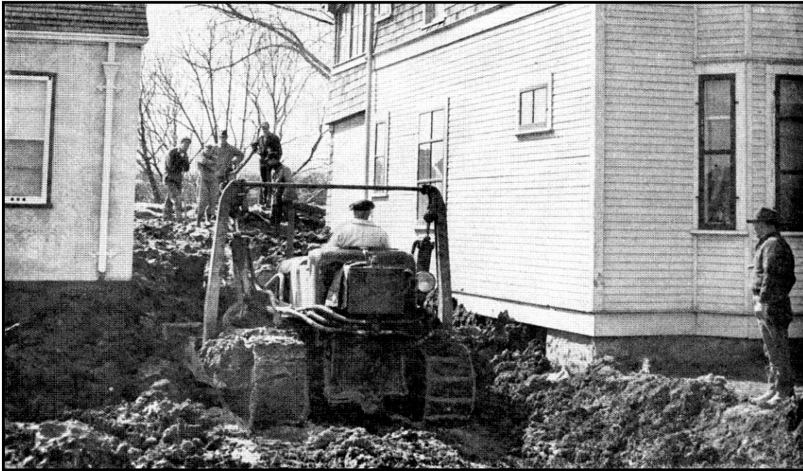
Left: A bulldozer packs dirt to bolster a sand-bag dike. Small storage building, garages, and sometimes even houses were sacrificed to allow builders a free hand. .
