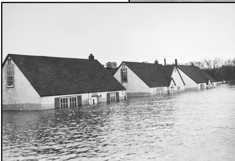
Left: A street of roof tops - stark evidence of the River's destructive flood waters. — over 1900 houses were flooded over the first floor.
