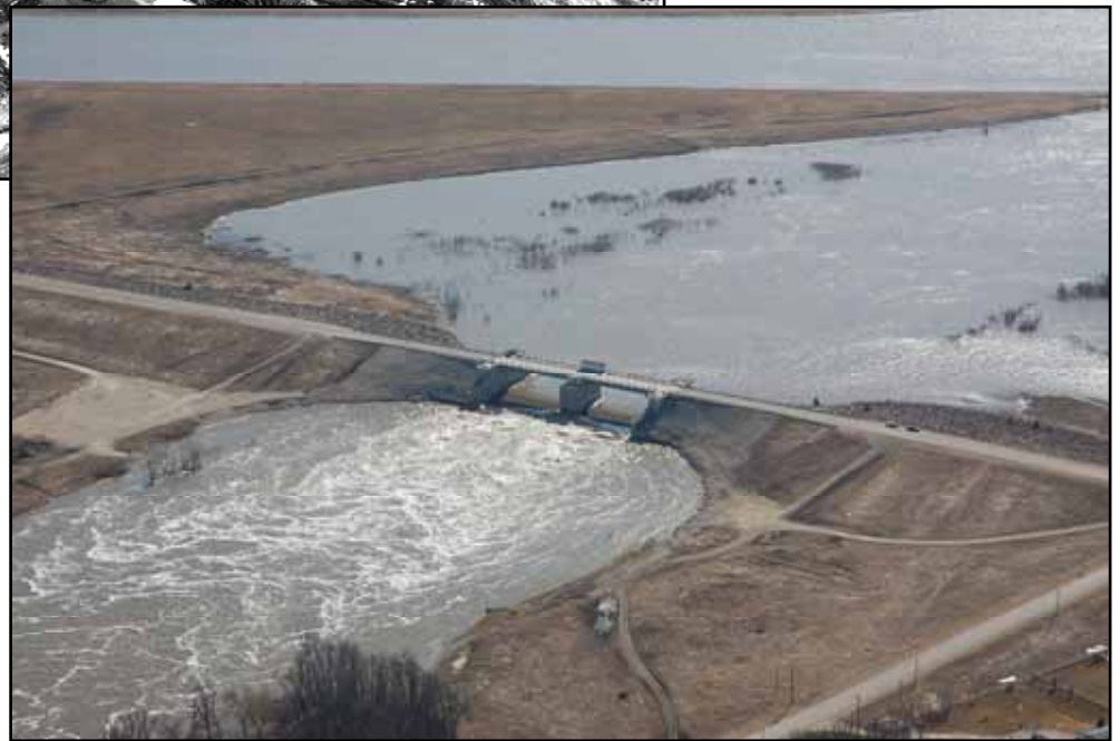
Right: The Red River Floodway inlet control structure in operation.
