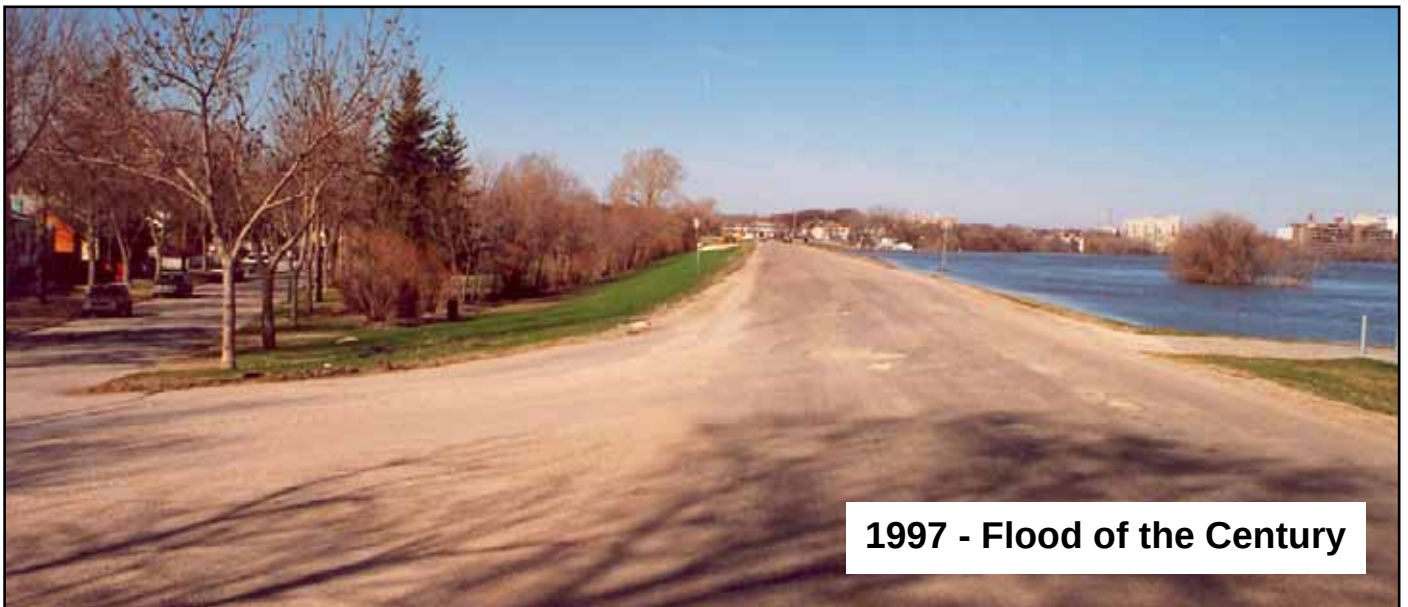
Below: Water lapping near the top of the permanent earthen dikes protecting the Wildwood district of Winnipeg.
