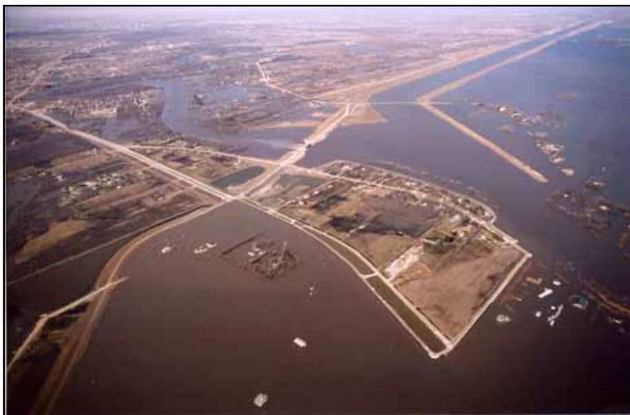
Left: The Floodway gate area during the 1997 flood. Note that Turnbull Drive is protected with its own ring-dike system. Note also the flooded low-lying areas north of the Floodway in St. Norbert. The Floodway was operating to its capacity and the excess water had to be directed into the city necessitating sandbagging in several areas of the city.
