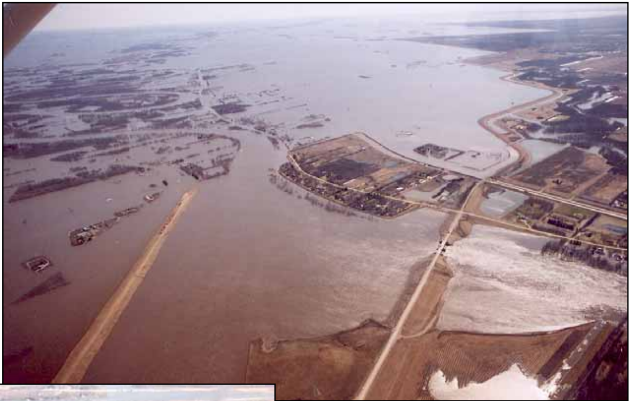
Above: An aerial view of the Floodway gate area, looking towards the southeast, and showing a section of the Z-dike which had to be strengthened and extended in a mere 72 hours to prevent floodwaters from inundating Winnipeg from the west.
